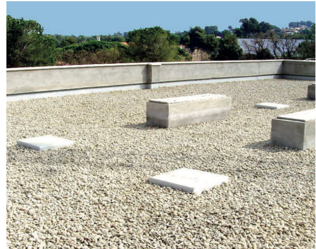
Example of a flat gravel roof
