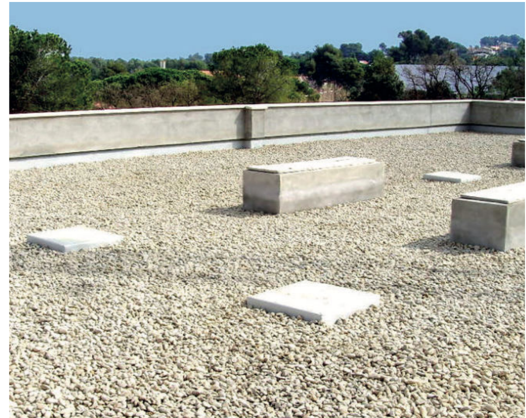
Example of a flat gravel roof
