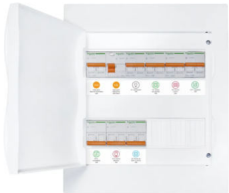
ELECTRICAL PANEL OF THE DWELLING
